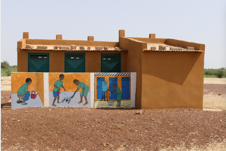
School latrine blocks
